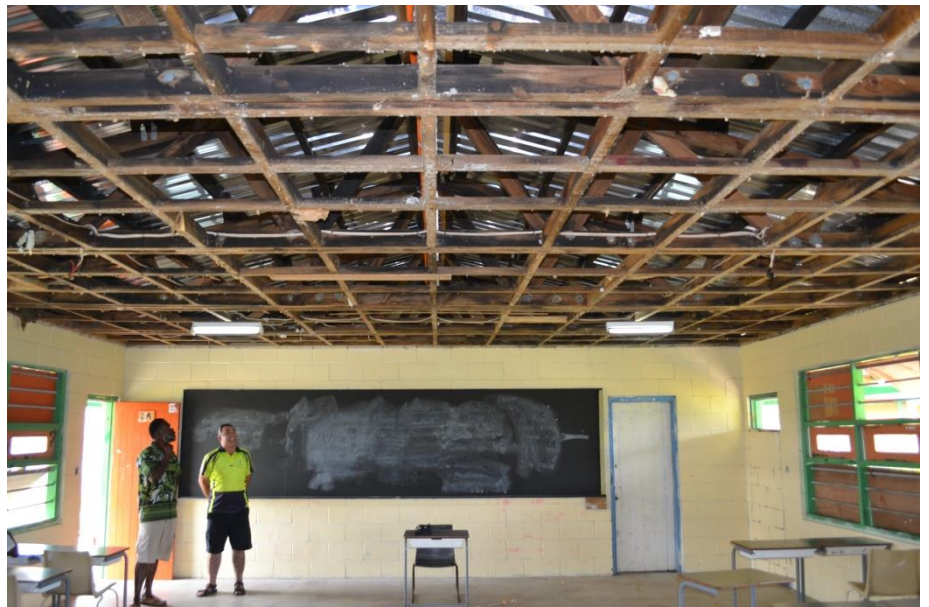
Neville Jones and Onesua College Principal Graham Kalmar inspect ceiling damage at the College following Cyclone Pam. PCANZ is funding these repairs.
