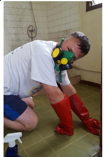
Richard cleaning tiles with Hydrochloric acid
