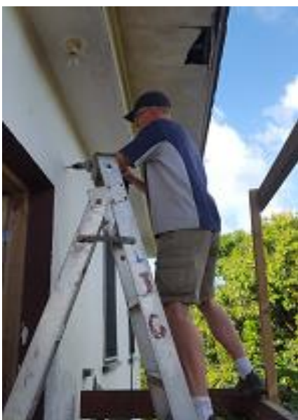
Simon building a veranda over the door
