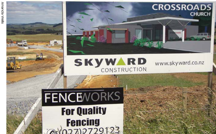
Construction of Crossroads' new church is well underway
